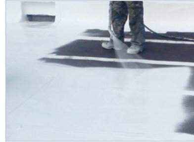
All protrusions in the roof were treated with a 3 course system (coating-fabric-coating) and received coating on the entire fixture. This ensured a watertight seal where the old system was vulnerable to leaks.
