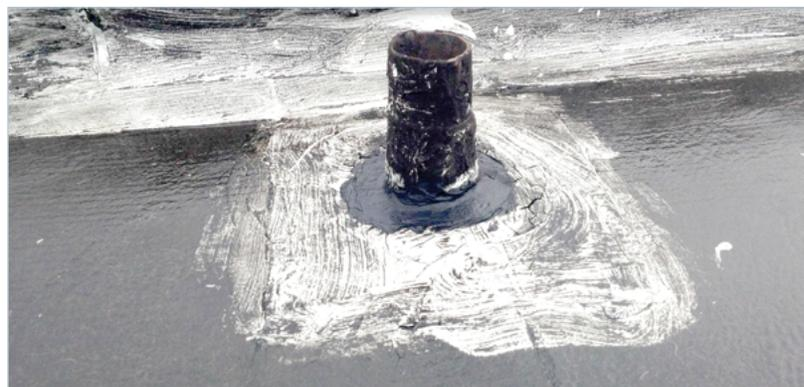
The previous roofing system, a smooth-surface built-up roof, had severe wear and tear around all protrusions and building edges. These areas were given a three-course silicone treatment of coating-fabric-coating to ensure a water-tight seal.
